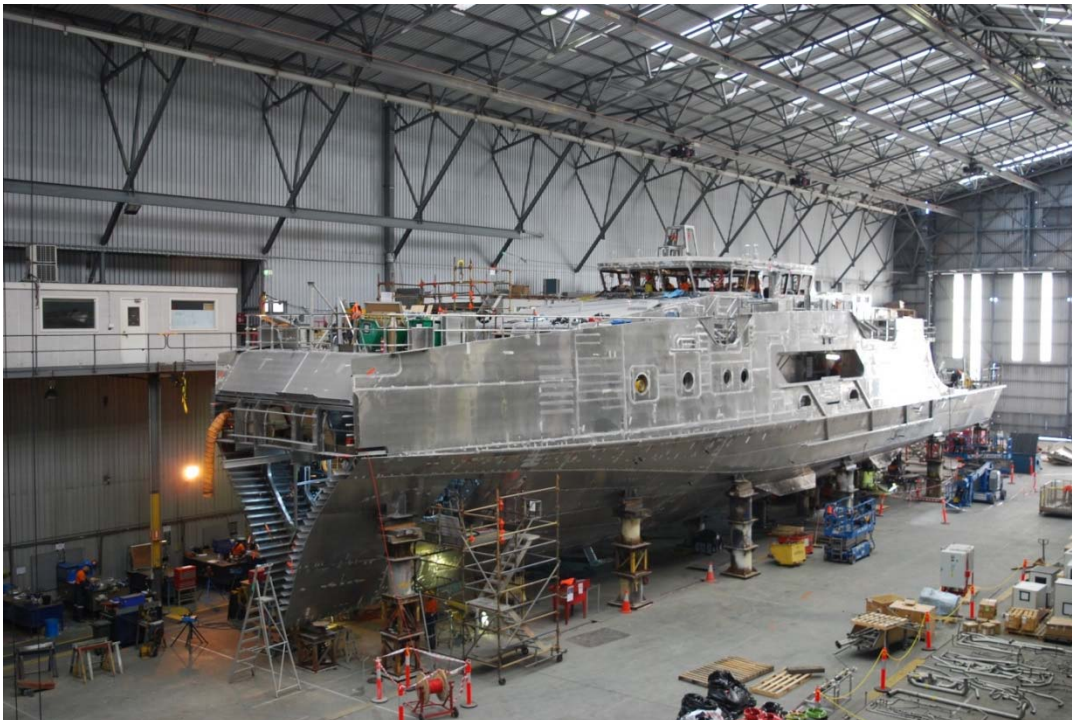
The ninth Cape Class Patrol Boat (Hull 380) under construction at Austal Australia
